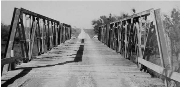
Lake Waco - 1959/Middle Bosque Bridge - End View
