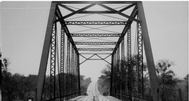
Lake Waco - 1959/South Bosque Bridge - End View
