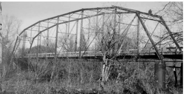
Lake Waco - 1959/McLennan Crossing Bridge - Side View
