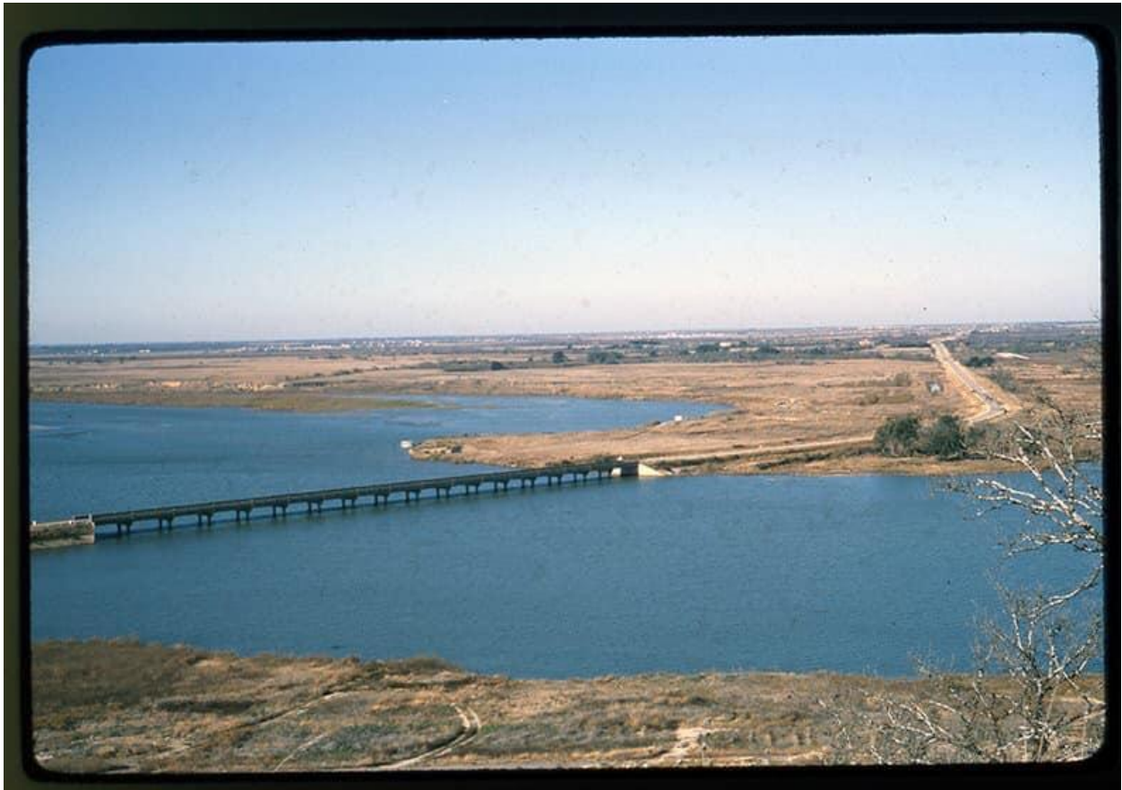
The old Highway 6 Bridge, 1964. Photo courtesy of The Texas Collection, Baylor University.
