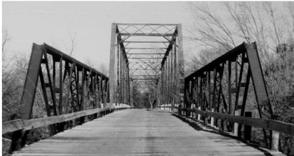
Lake Waco - 1959/DeHay Bridge - No Bosque End View
