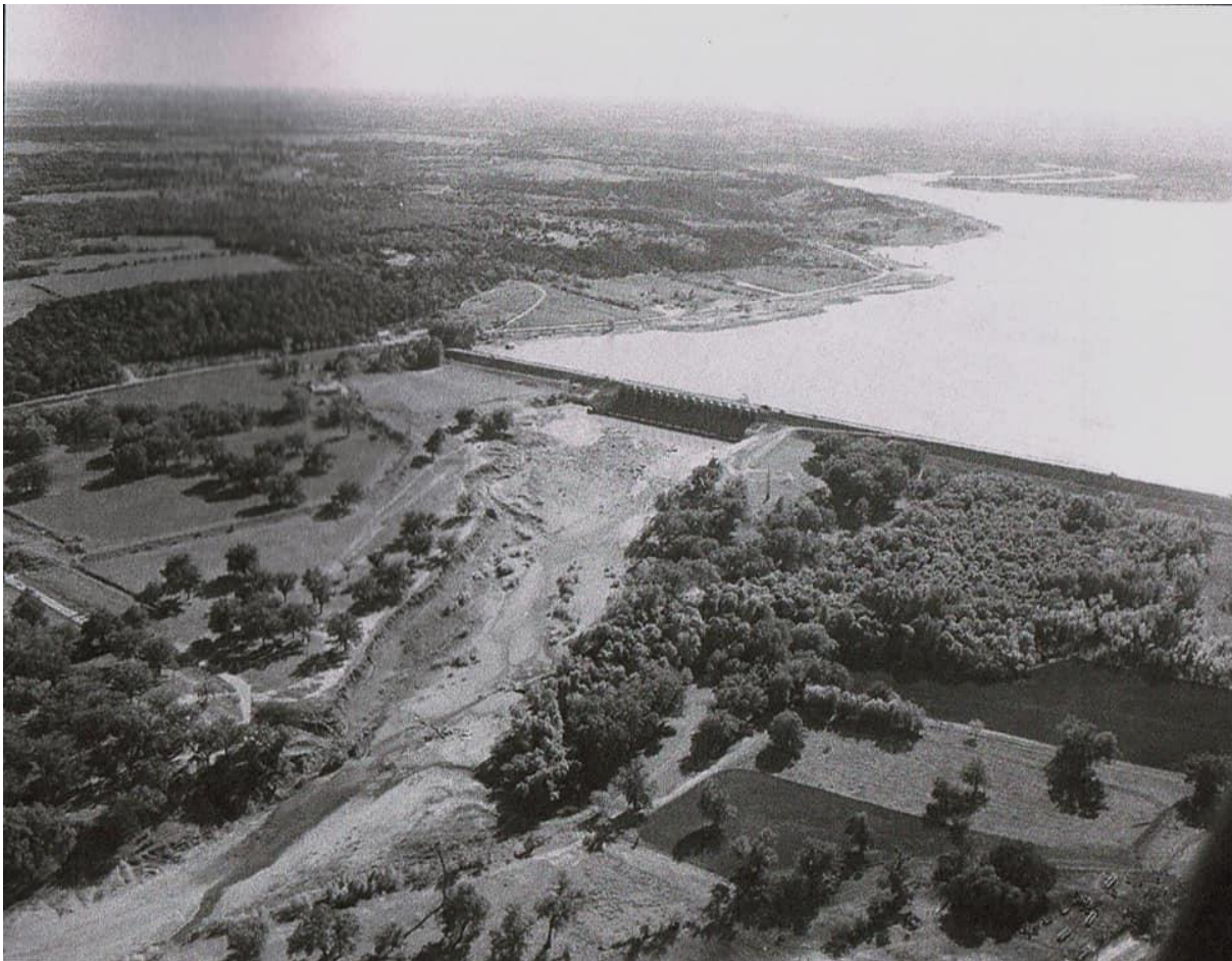
The 1930 Waco Dam, Waco on the left of the photo and the Waco Regional Airport area on the right. Photo from the book “Waco, Texas: A History and Photographic Retrospective of the Late Forties Through the Mid-Fifties” (2009) by William Lannie Burdsal, Jr.
