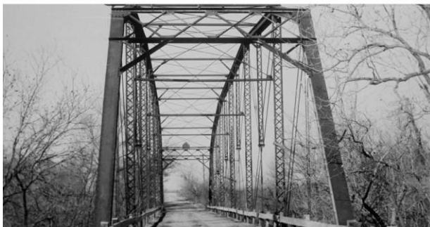
Lake Waco - 1959/McLennan Crossing Bridge - End View
