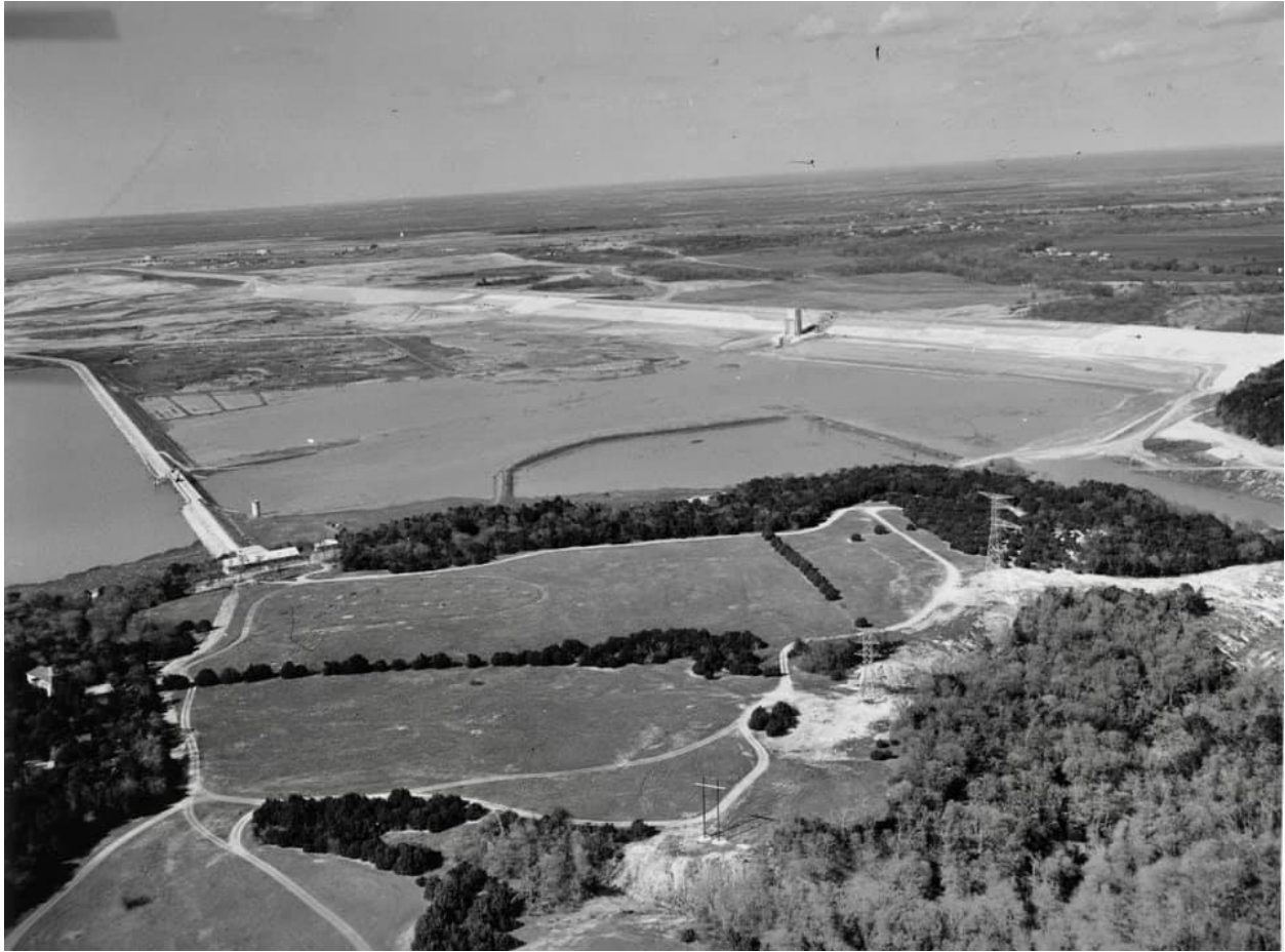
The Old and New Waco Dam, January-February, 1965. Photo by Windy Drum. This photo was taken by Windy Drum, 1965. Copyright by James Jasek, and is used with his permission. Do not share this photograph without the attached photo credit and copyright information.
