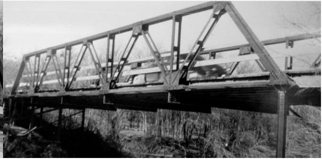
Lake Waco - 1959/Hog Creek Bridge - Side View
