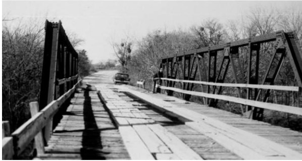
Lake Waco - 1959/Hog Creek Bridge - End View
